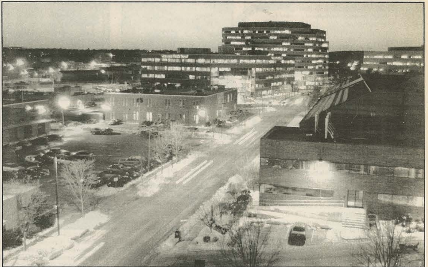
Cambridge Park Drive looking west to Spaulding & Slye's 1980s office park
