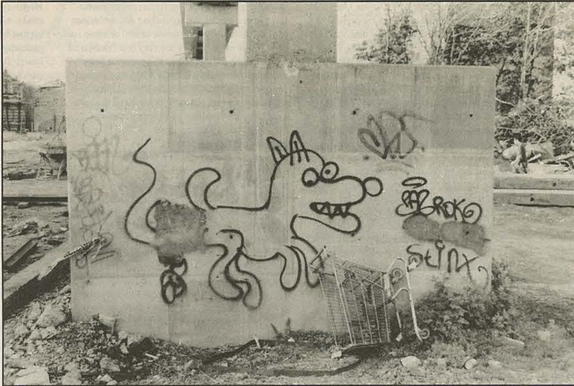
Public comment on the new bridge abutment under Alewife Brook Parkway
