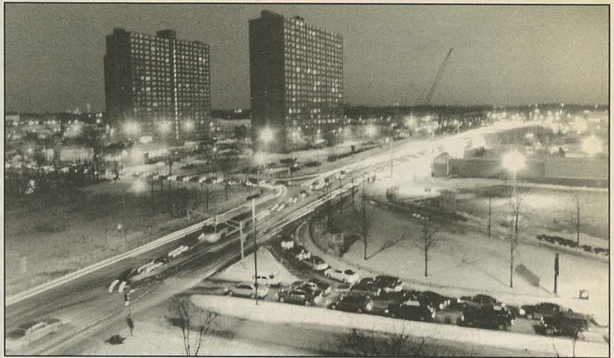
Alewife Brook Parkway, looking south
