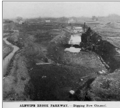
ALEWIFE BROOK PARKWAY. — Digging New Channel.
