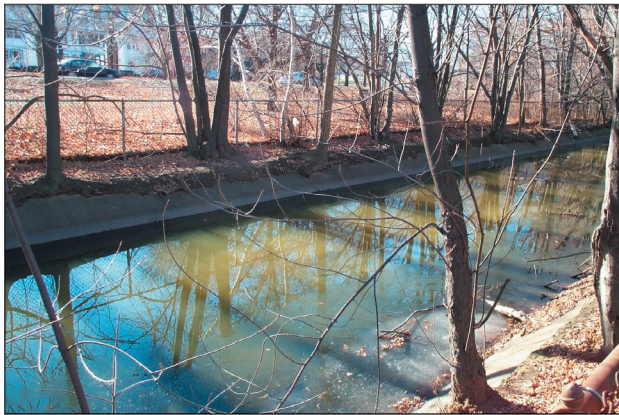
FIGURE 57. The Alewife Brook flows in a concrete-lined, straight channel in this area.
