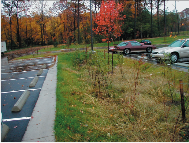
FIGURE 29. A biofiltration area in a parking lot.
